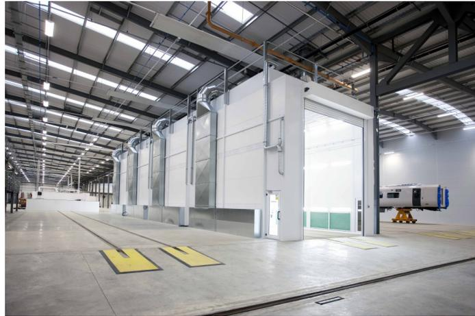
An iSystem touch control pre-programmed with bake cycles was fitted to operate the spray booth. Hitachi Rail can now be confident of ensuring paint jobs are not over or under cured as operators can select from a list of coatings used and the most efficient cure profile is automatically executed. The iSystem also balances the air pressure within the cabin ensuring adherence with COSHH regulations.
